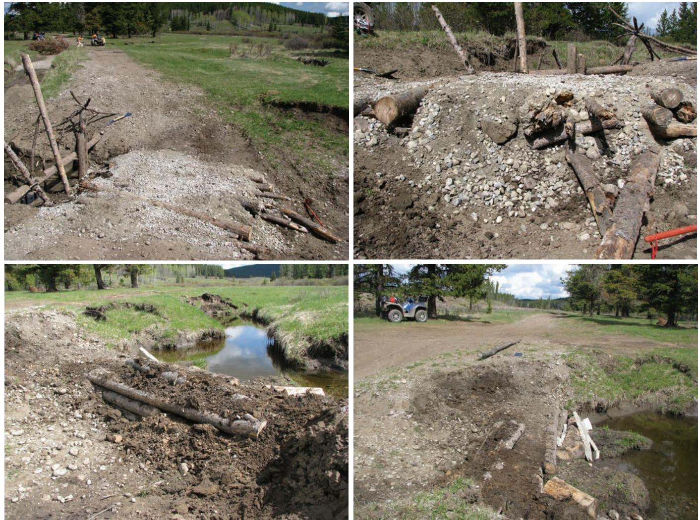
Our largest project was behind the gravel pit at WP# 109. During the May Long Weekend this hole was identified by a rider who got so stuck that his quad was jammed between the wall of the banks. Using only shovels, picks, buckets and our quads the crew filled, transferred and dumped over 100, 10 gallon buckets to fill these holes.
